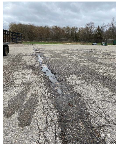
Figure 2 – Existing asphalt conditions at the time of investigation.
