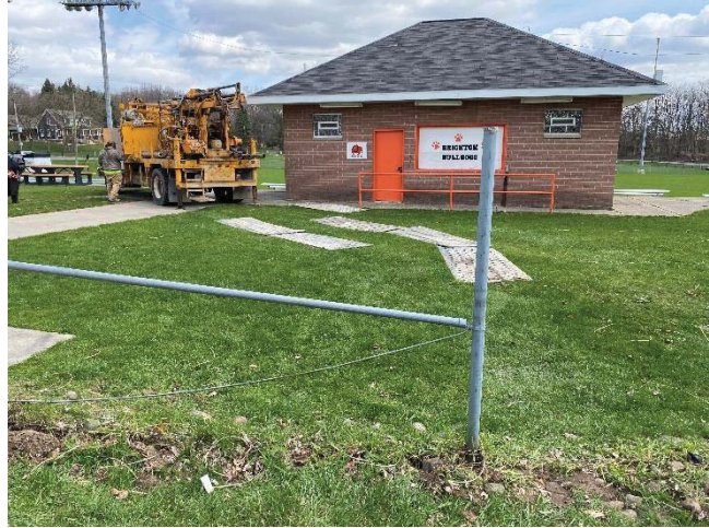
Figure 2 – Access with fence section removed and mats in place
