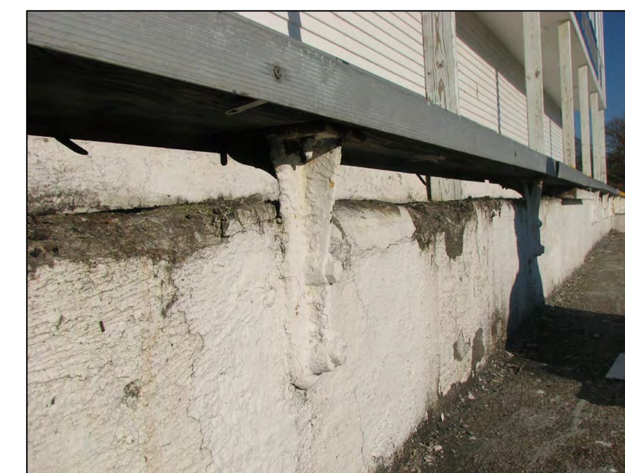
EXISTING SEAT BRACKET SCALE: NO SCALE (FOR INFORMATION ONLY)
