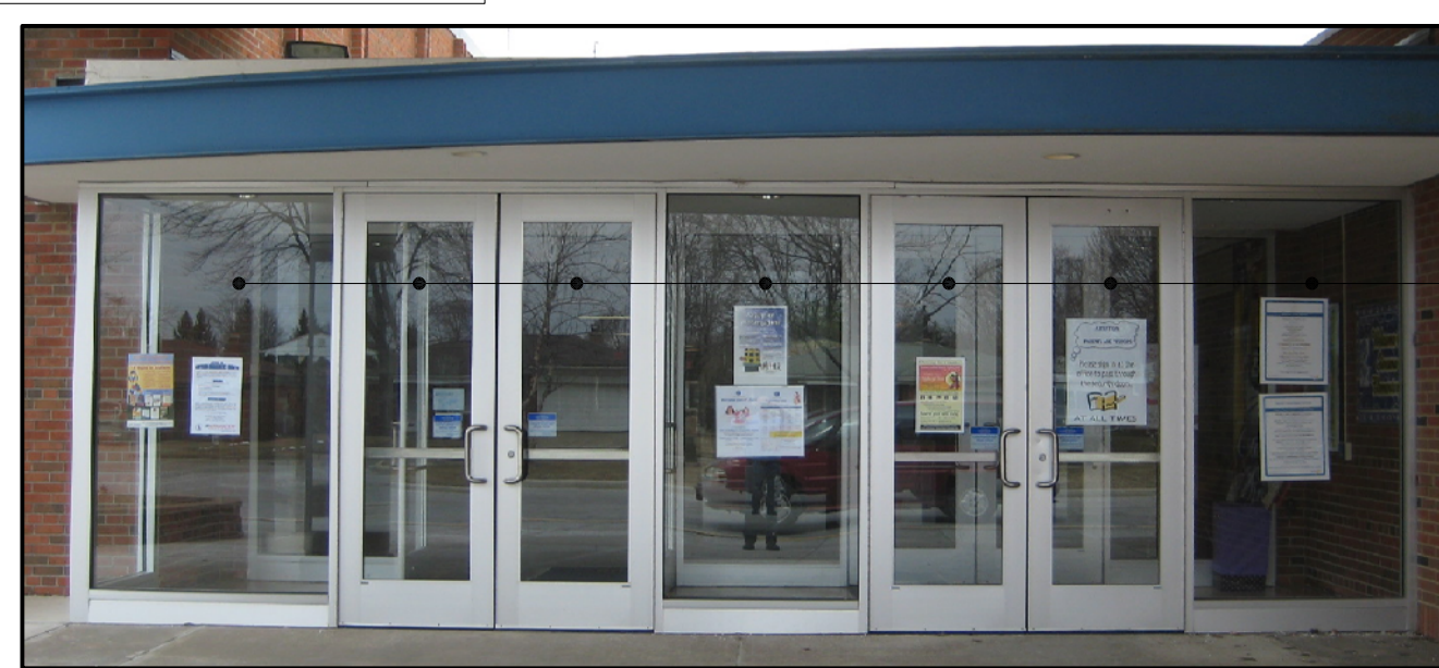
NOTE: PHOTO SHOWN IS EXTERIOR- FILM TO BE INSTALLED AT INTERIOR SIDE OF GLAZING APPROXIMATE GLAZING AREA: 188 SF
