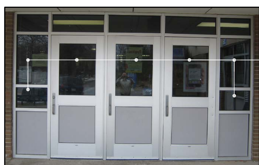
NOTE: PHOTO SHOWN IS EXTERIOR- FILM TO BE INSTALLED AT INTERIOR SIDE OF GLAZING APPROXIMATE GLAZING AREA: 60 SF
